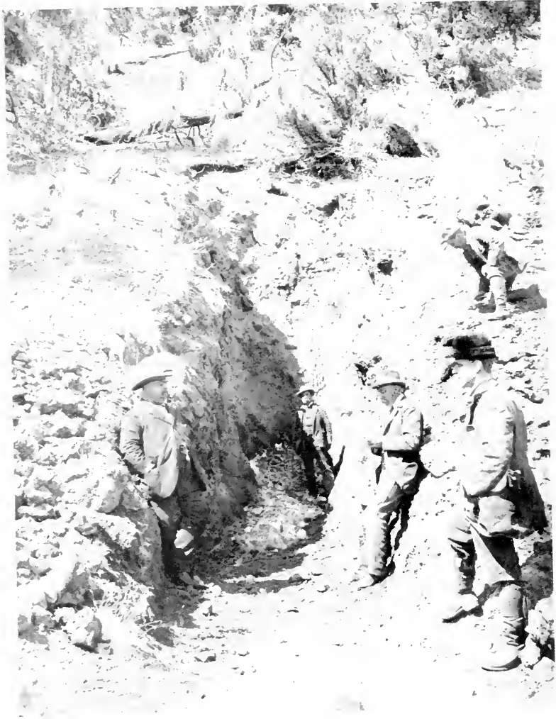
OPEN CUT IN SOLID IRON ORE.
